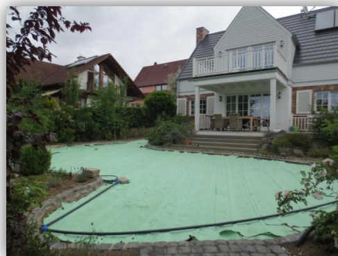
Installed iMat cut to the area to be irrigated
