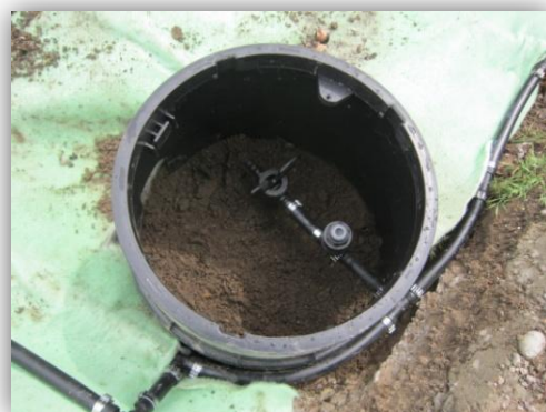
Additional small valve box with shut-off valve and air/vacuum relief valve
