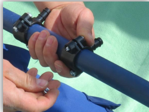
Installing the clamp saddle
