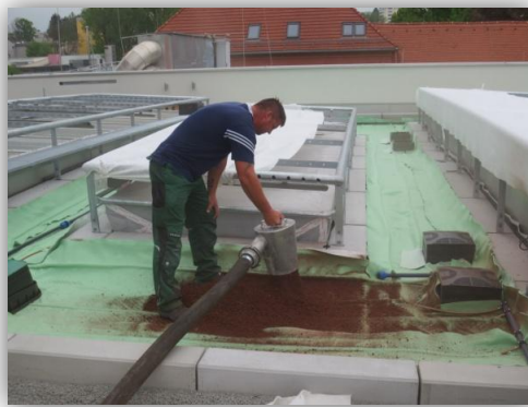
Blowing up substrate
