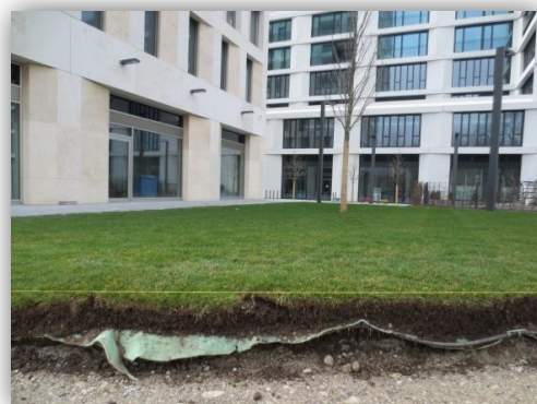
Subsurface installation of iMat
