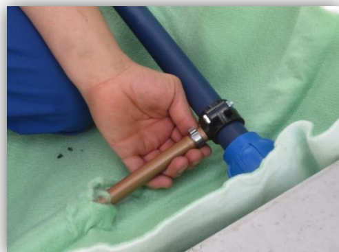
Connecting the dripline and securing with a pipe clamp
