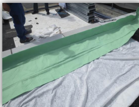
Lay the side of the matting strips right up to the edge or even pull them up to the side on the edge to prevent the formation of brown edges.
