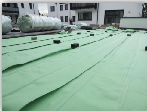
Lay iMat strips with lateral overlap
