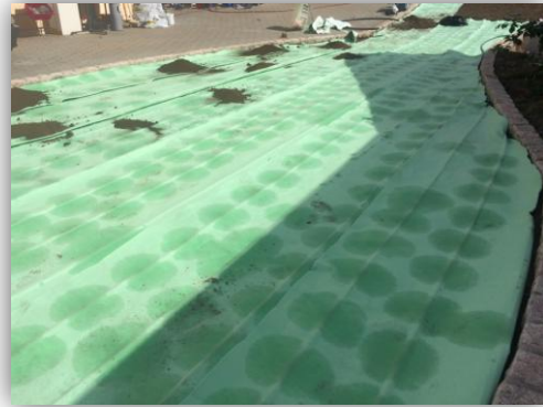
Test operation before backfilling
