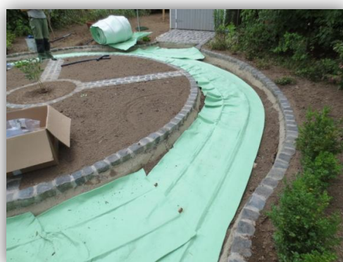
Installing the iMat in curves
