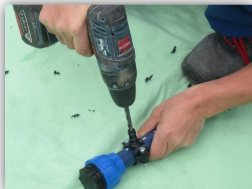
Drilling the PE pipe open through the clamp saddle
